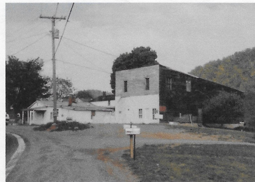
St. Clair Brothers Garage (later photograph, with sign painted over). Guy was born in the second-floor apartment. The building has since been demolished.
