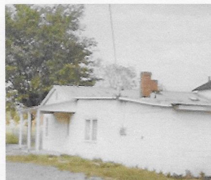
Filling station with add-on rooms
